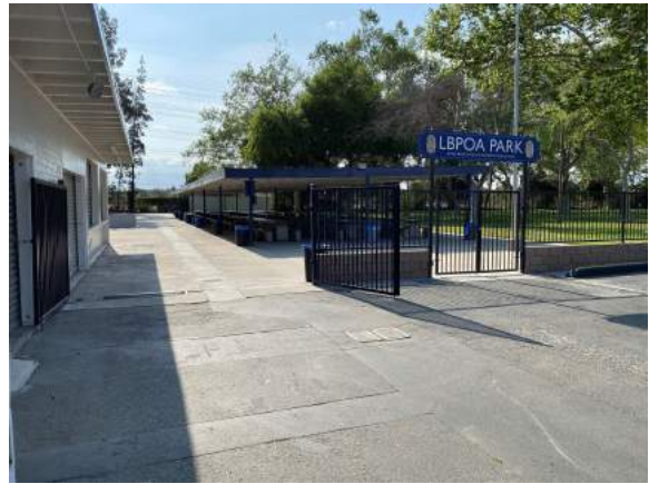
VEHICLE ACCESS GATE
